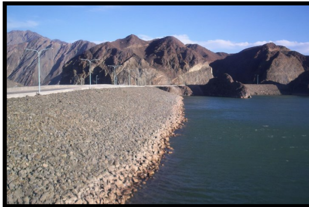
Figura 12: Defensa ribereña Dique
