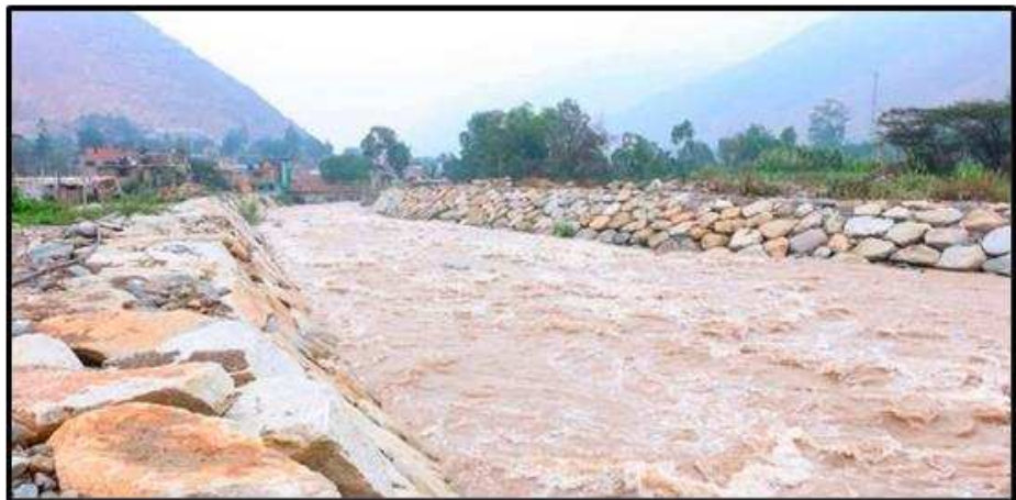
Figura 8: Defensa ribereña enrocado
