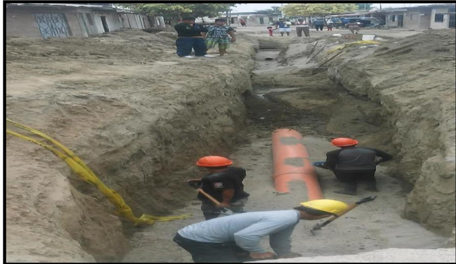
Figura 5: Colector Principal Ø 16” PVC
