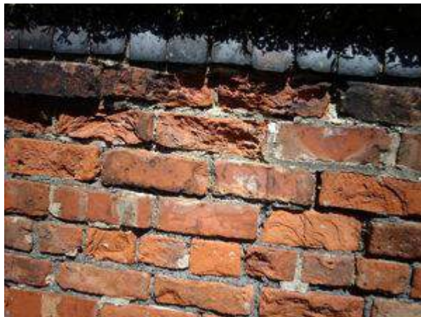
Figura 8: Erosion
