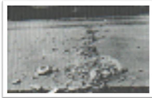
*Figura 8:* Blow Up / Buckling.
