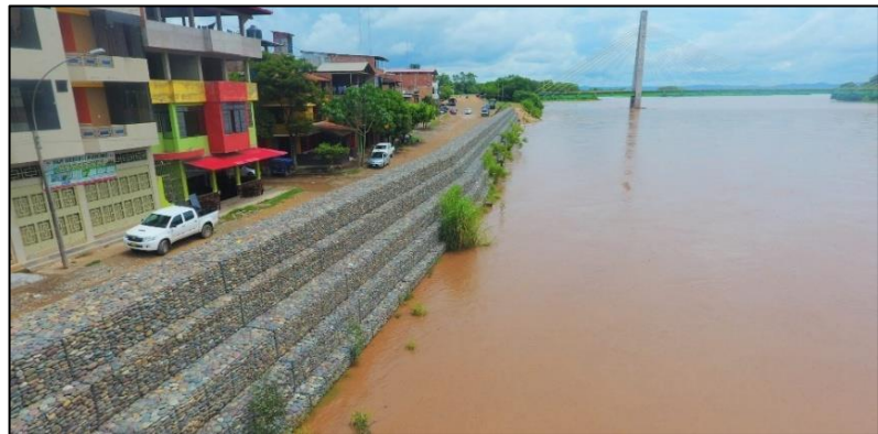
Figura 13: Defensa ribereña río Huallaga
