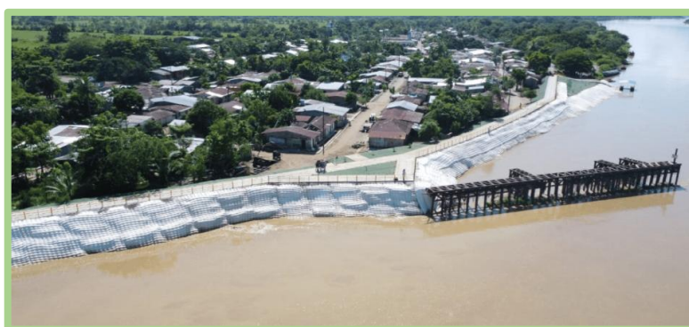
Figura 31: Defensa ribereña geotextil
