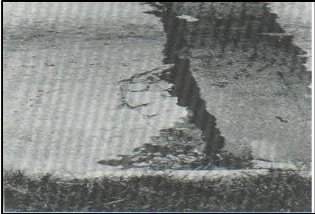
Figura 9: Blowup / Buckling severidad media
