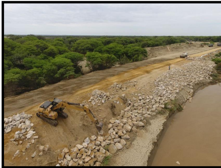
Figura 6: Defensa ribereña enrocado
